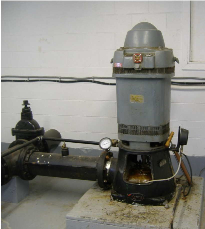
VERTICAL TURBINE LINE-SHAFT
